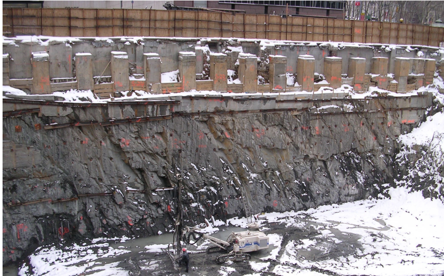
Figure 2: Excavation picture at subgrade along 6 th Avenue
