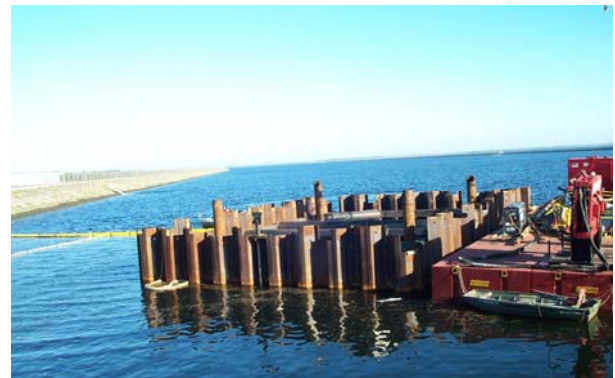
Figure 10: Cofferdam during construction
